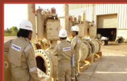
On-Site Valve Repair
