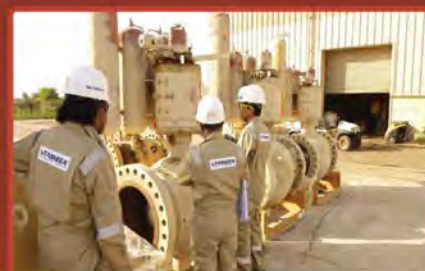
On-Site Valve Repair
